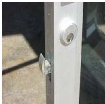
Commercial door with a type of mortise lock installed.
