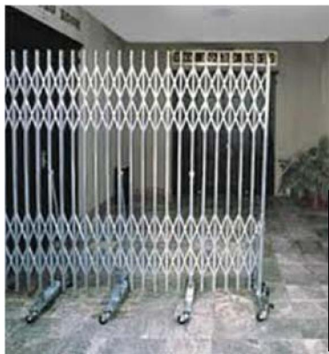
Limiting access to hallways and classrooms during after-school activities can be accomplished by a barrier such as a scissor gate.
